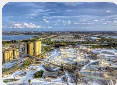
Pennsuco cement plant, USA
