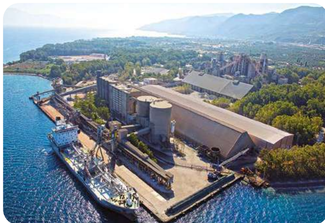
Patras cement plant, Greece
