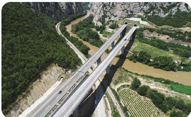
Demir Kapija – Smokvica Highway, section of Corridor 10, N. Macedonia
