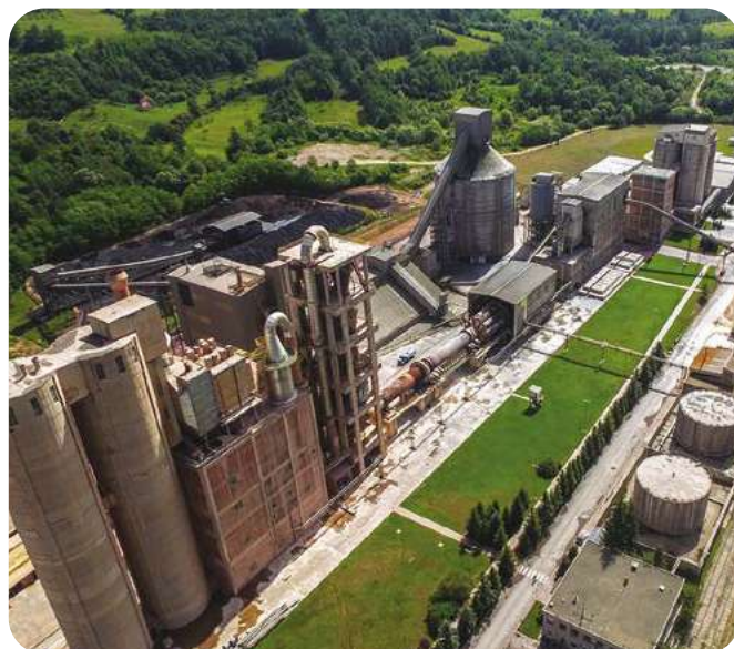
Kosjeric cement plant, Serbia
